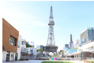
Chubu Electric Power MIRAI TOWER (former name: Nagoya TV Tower)
