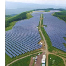
Nagato Farm Mega Solar Power Plant (Nagano)
